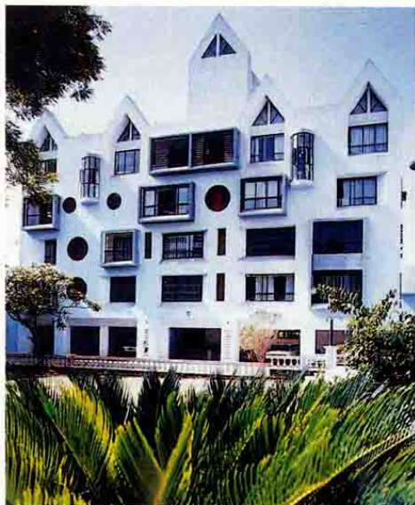
Konark Estate, Pune. A restrained composition that responds to its context. The beautiful sloping roof of a nearby bungalow prompted Contractor to adopt pitched roofs in this building, one of his earliest.
