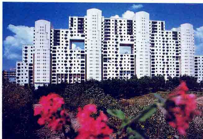
Rear view showing the four staircase blocks.
