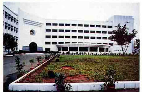
Bharat Petroleum, Bombay. The form and function again dovetailed quite well in the projecting semi-circular dining halls that maximize the view of the garden.
